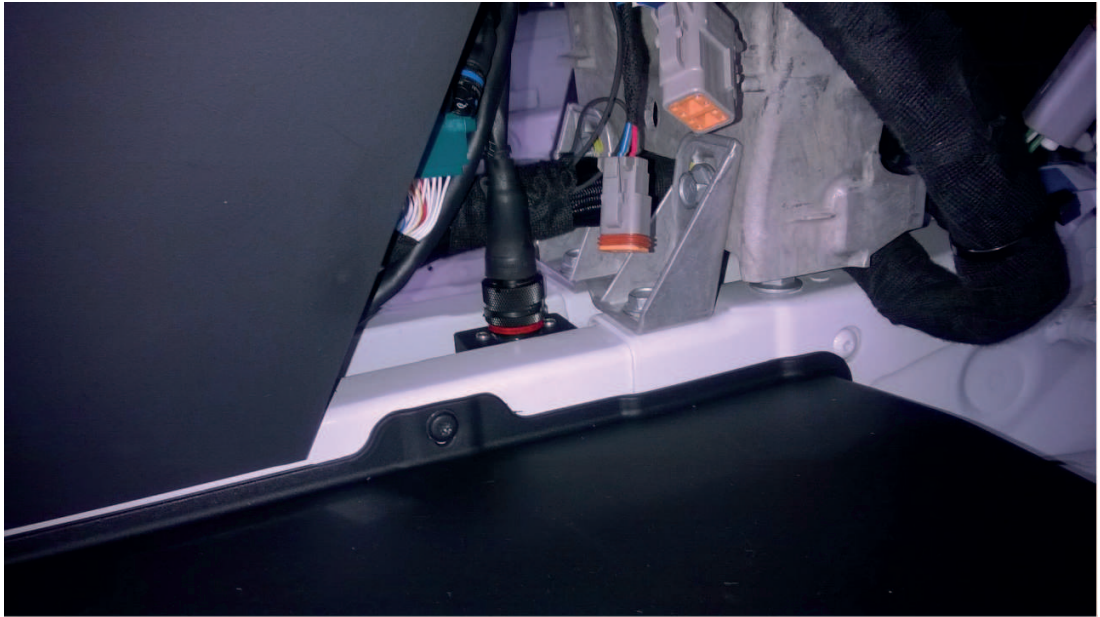
Figure 5.2: Wheelspeed signal splitter with wiring loom plugged in
